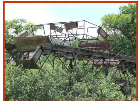
Hanging Flume construction (photo by Gen9Productions)
