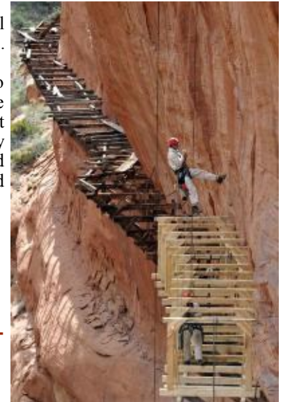
Hanging Flume construction photo by Gen9Productions
