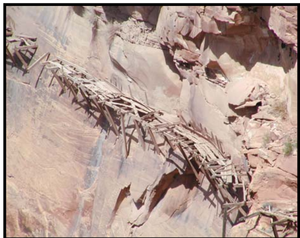
Figure 2. Section of the Flume showing deteriorated condition in 2002 (near location of arrow in Figure 1).
