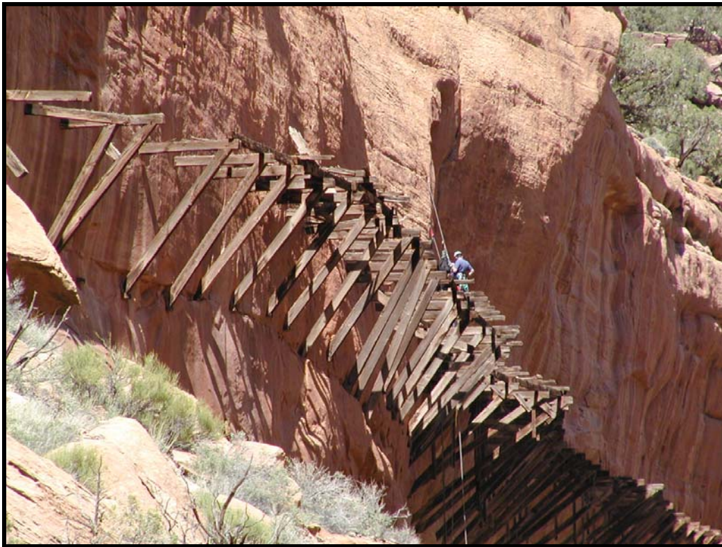
Figure 4. Engineers and industrial climbers rappel to a relatively intact section of the Hanging Flume.
