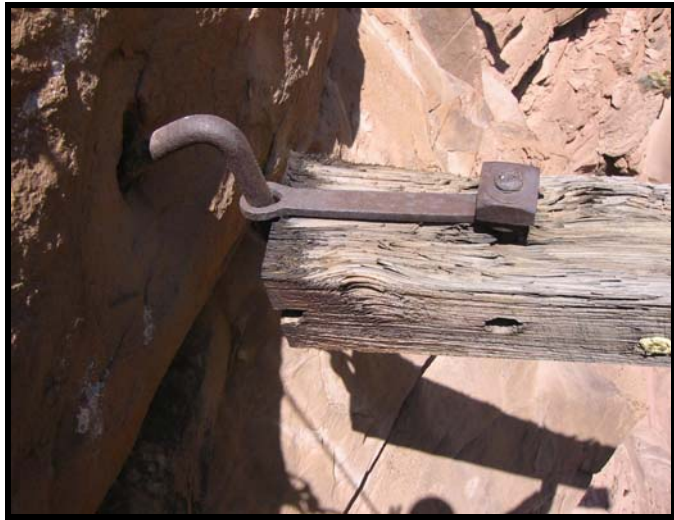
Figure 8. Anchor rod configuration using a flat strap washer.
