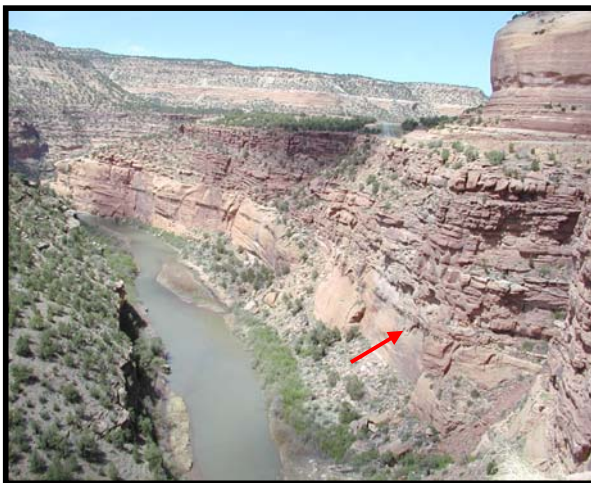
Figure 1. View of the Hanging Flume above the Dolores River. The arrow points to only one of the Flume segments which can be seen in this photo.
