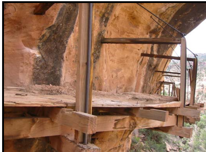
Figure 12. An example of type D brackets found in one segment of the Hanging Flume.
