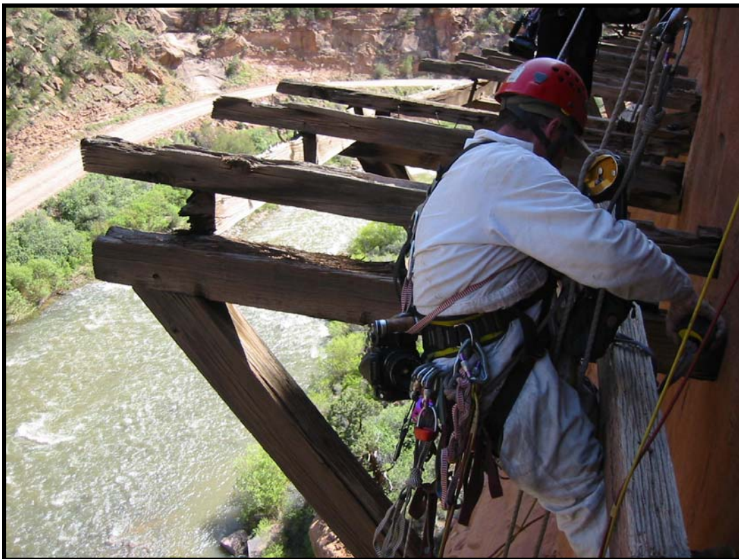
Figure 5. Engineers and industrial climbers measure and document the Hanging Flume at a drop site along the San Miguel River.
