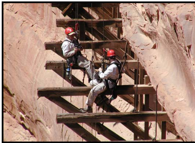
Figure 10. An example of type C brackets in a segment of the Hanging Flume.
